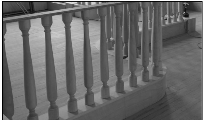
Reconstructed rails and spindles
